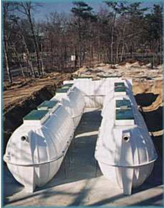
View of a Cromaglass unit during installation.
