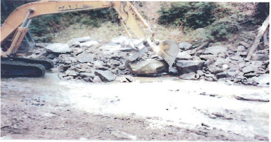
c) Placement of boulders at Site 11
