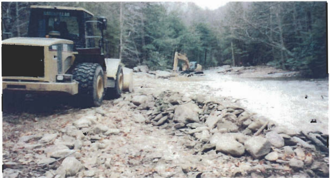
b) Building of structures at Site 19
