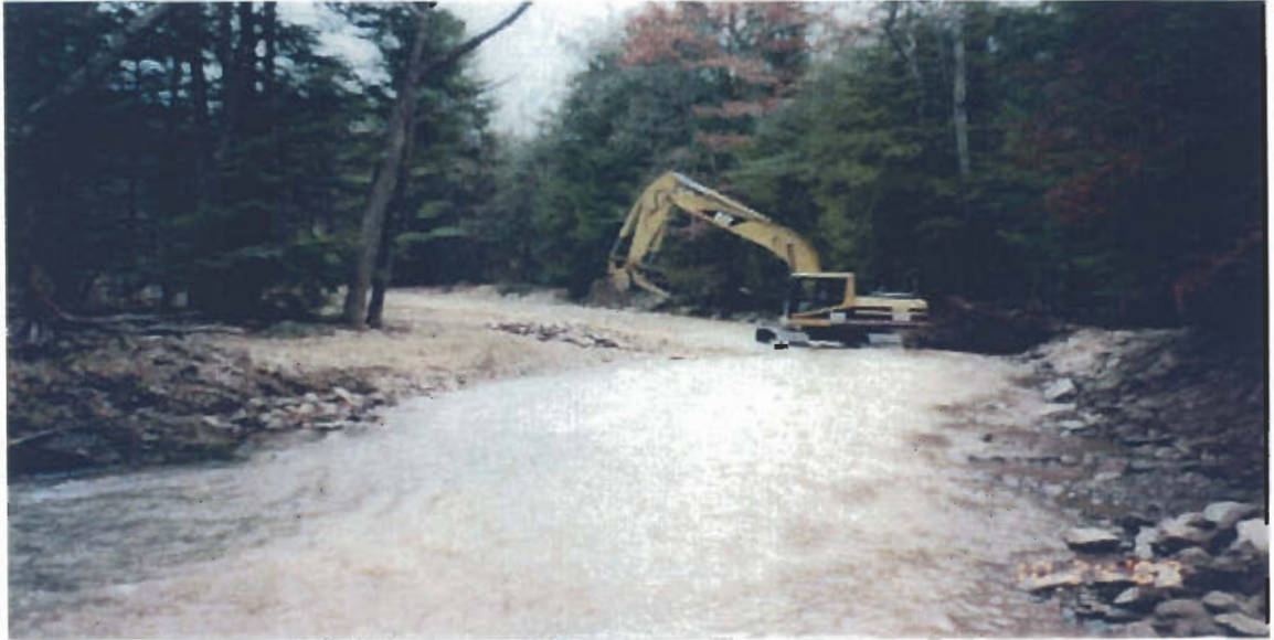
a) Machinery preparing to build structure near Site 16
