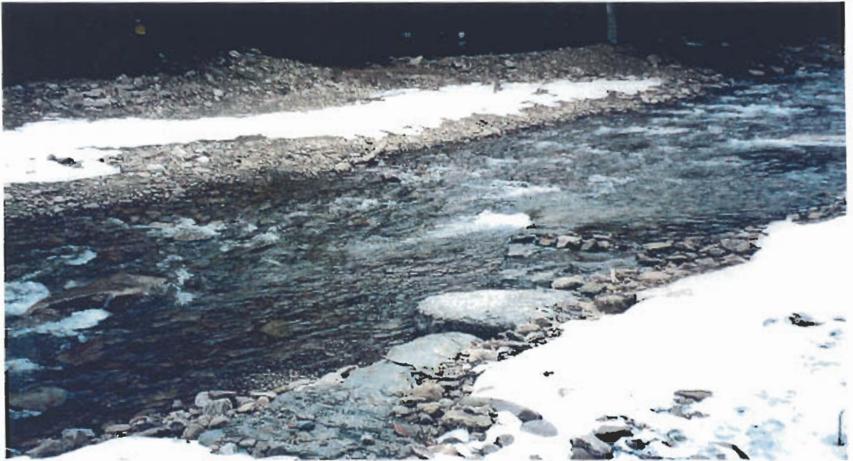
a) View from right bank looking slightly upstream at J-hook structure at Site 16
