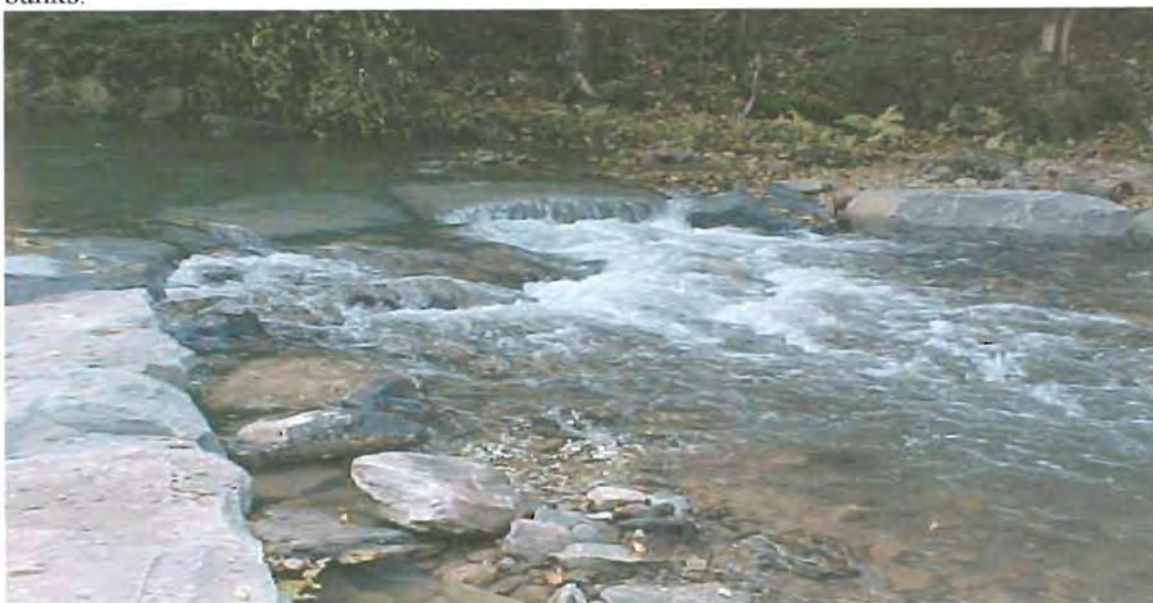
Figure D. A truncated cross vein rolls water to the center of the stream, protecting the banks.
