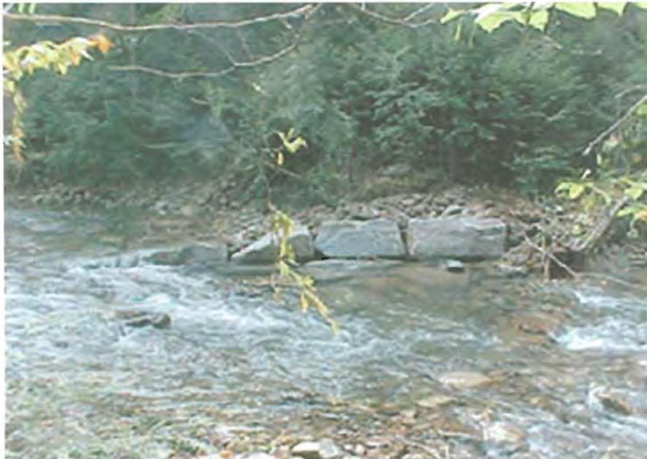
Figure C. A J-hook vein provides erosion control and some great trout habitat.
