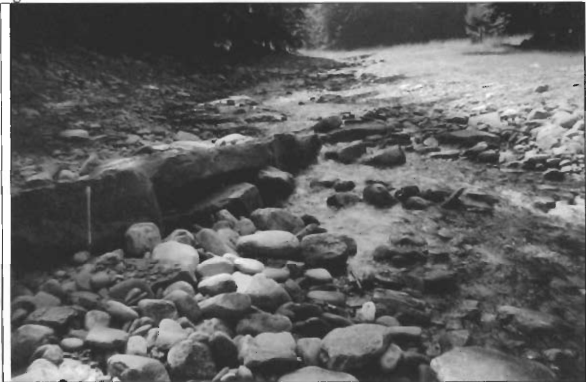
Figure 6 J – Hook Structure Under Normal Conditions
